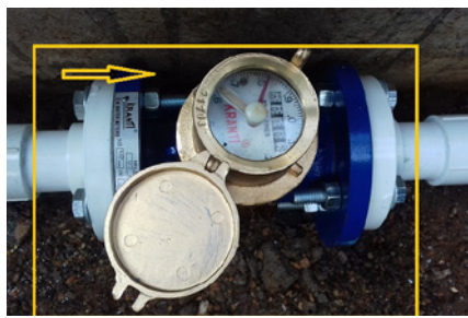
Installation of Flow meter at specific areas for water mass balance
