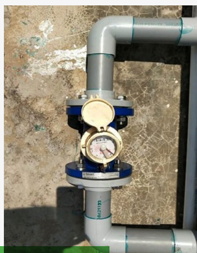
Water flow meters installed in various units for continuous monitoring of Fresh Water and Waste Water
